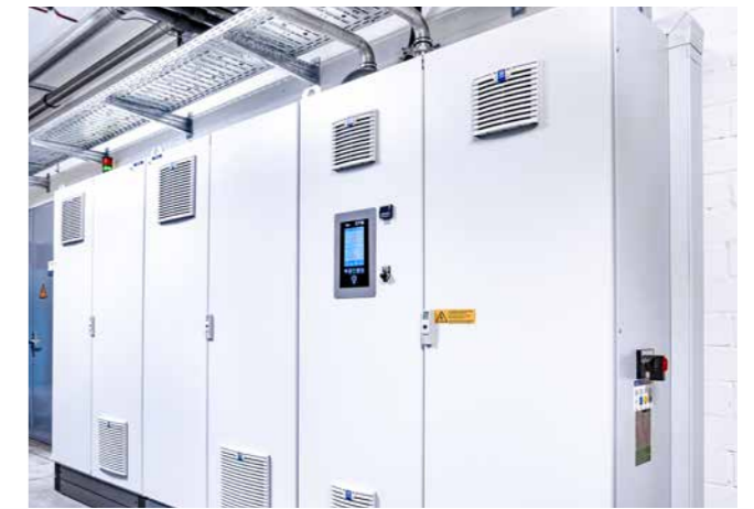
Electric control cabinet Control of temperature and humidity
